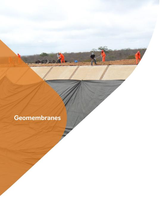
Geomembranes are thick plastic linings (0.75 to 3.0 mm) whose function is containment or waterproofing, preventing the passage of liquids and vapors. Due to growing environmental awareness, combined with regulations, their use is growing, especially in the infrastructure, construction, and agricultural sectors.
